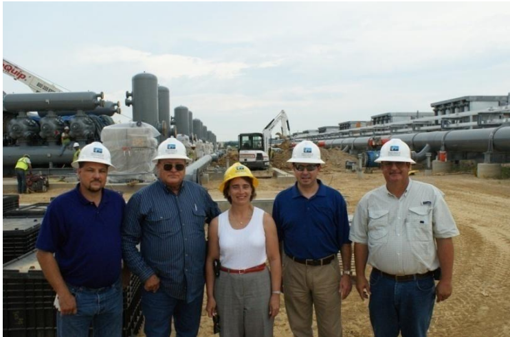
Pictured: Sen. Lincoln (center) tours the Russell Compressor Station with FEP personnel.
